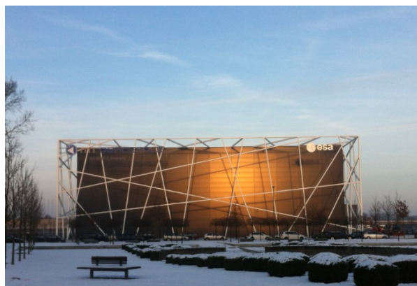
Figure 23. MTA facilities in Bremen
