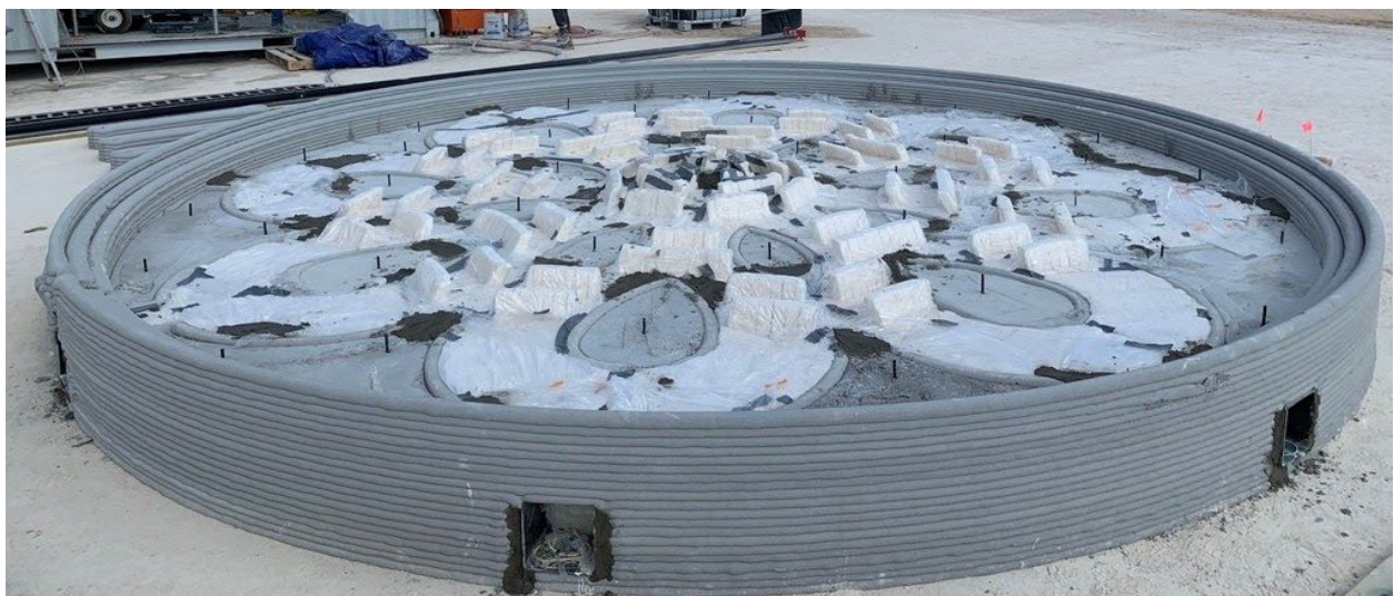
Fig. 14 Foam and viscous concrete placement prior to the final cast fill
