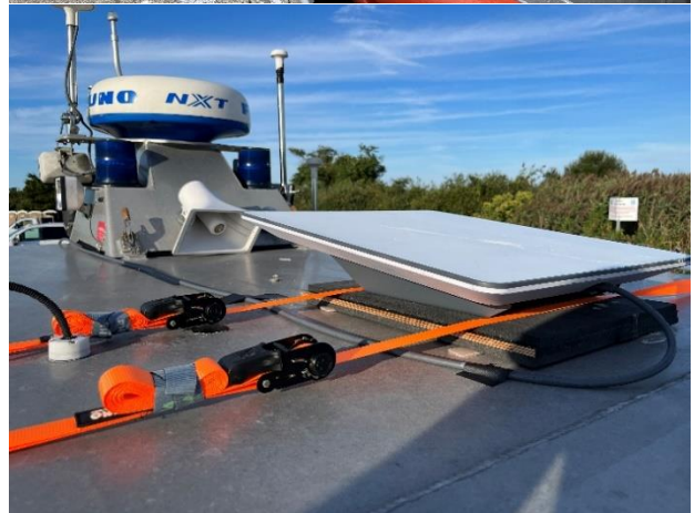
Figure 3. Starlink antenna installed on the RDC’s RB-S (Source: U.S. Coast Guard).
