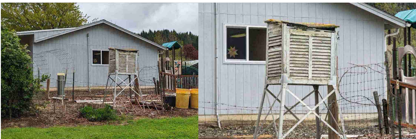
CRS placement at rear of Cooperative Observer's residence at Elkton, ID. Note the deterioration of the CRS, including rot, mold, and peeling paint. Observations are still taken daily here. Source: Anthony Watts.
