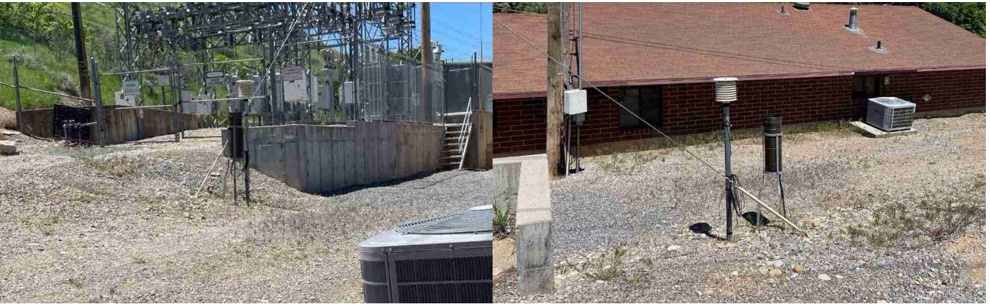
MMTS placement at USHCN station in Spanish Fork, UT. Note the a/c unit and the power substation. Also note the proximity of the roof, due to the thermometer's elevation. The location is at a power generation facility. Source: Steve Randle and Ron Broadway.
