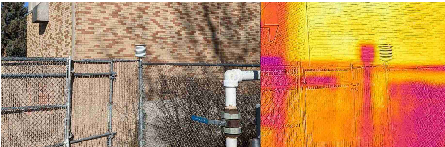
Visible and infrared photos of MMTS placement near large sunlit wall and electric power generation plant at Dillon, MT, USHCN Station at Western Montana University. Source: Anthony Watts.
