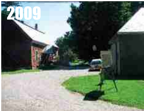
Enosburg Falls, VT , adjacent to driveway, nearby building. RATING = CRN4
