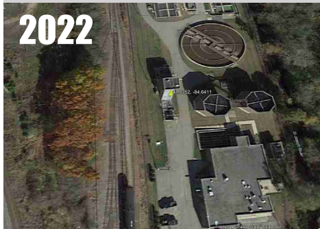
No change in location. Unable to ground survey. RATING = CRN4
