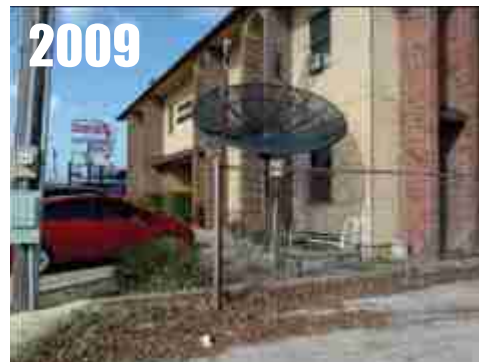
Lampasas, TX , next to sidewalk, near satellite dish, road, parking lot, building. RATING = CRN5
