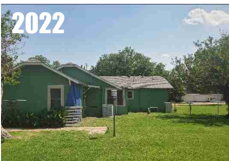
Location moved, but now near sidewalk and A/C unit, building. RATING = CRN4
