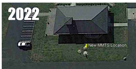
Same location at city WWTP, but MMTS moved to a better location over grass in front of office. Better site, but still too close to road and the building. See markers. RATING = CRN4
