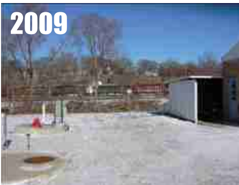
Logan, IA, nearby building, concrete slabs. RATING = CRN4
