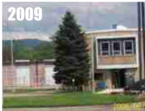
Uniontown, PA , nearby building, road, parking areas. RATING = CRN4
