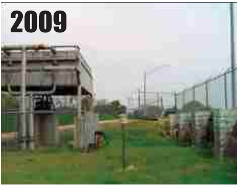
Red Cloud, NE , on premises of city power plant. Nearby brick wall, structures. RATING = CRN4
