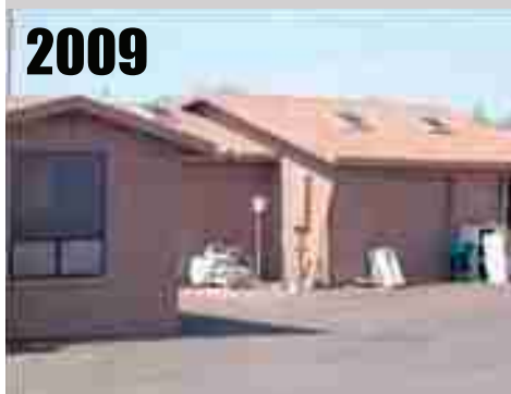
Wickenburg, AZ , adjacent building, parking lot, accumulated junk. RATING = CRN5
