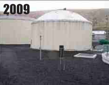
Heppner, OR , MMTS in a sea of dark crushed rock, at city WWTP. RATING = CRN5
