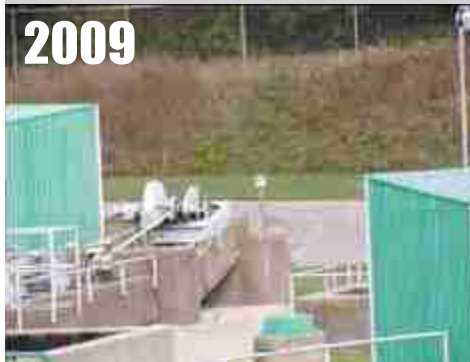
Napoleon, OH , over concrete, near wastewater Tank at WWTP. RATING = CRN5
