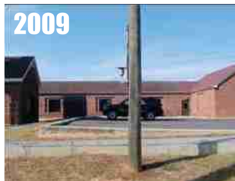
Orangeburg, SC , nearby metal coverings, parking lot, building at WWTP. RATING = CRN4
