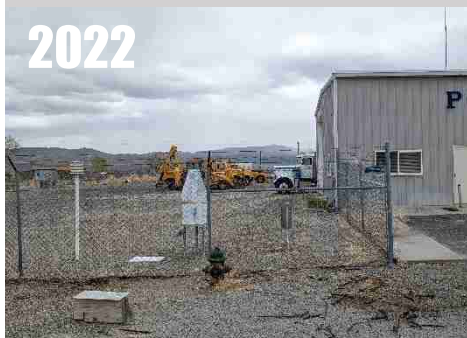
Closed, then moved to an industrial area, worse location. RATING = CRN5
