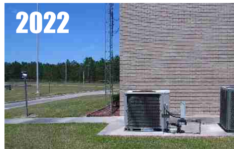
No Change. However, MMTS is dirty/discolored and needs maintenance. RATING = CRN5
