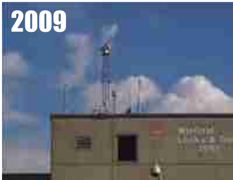
Winfield Locks, WV , MMTS is up on the roof. RATING = CRN5
