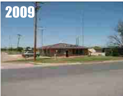
Haskell, TX , between road and parking lot, nearby building. RATING = CRN4
