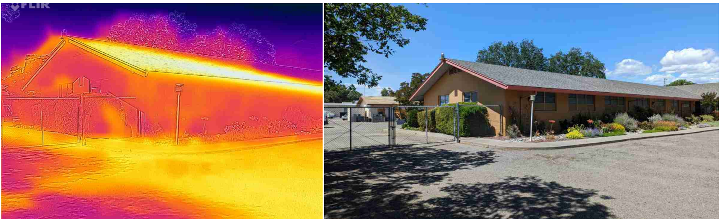
Visible and infrared photos of MMTS placement near roof and large parking lot at Woodland, CA, GHCN Station at the Yolo County Office of Weights and Measures. Source: Anthony Watts.
