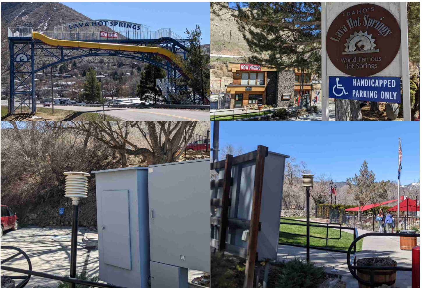
MMTS placement at Lava Hot Springs, ID, GHCN station. This is a tourist attraction where the MMTS sensor was placed into a natural hole in the ground where hot water for bathing and swimming emanates from the natural depression in the ground. In addition, the MMTS is next to a parking lot, a stone wall, and a sidewalk, all of which are heat sinks. The nearby electrical panel may generate heat. Because the MMTS is below average ground level in the natural depression, it is also wind-sheltered, which prevents atmospheric mixing and thus will not be representative of temperatures in the nearby landscape. Source: Anthony Watts.
